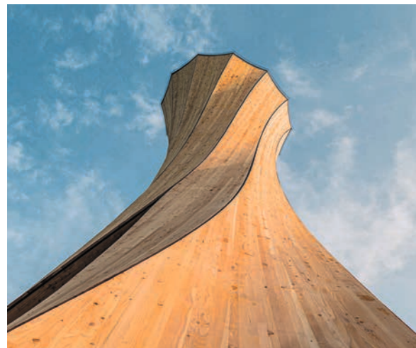
Known principles put to new use: when moist wood dries, it contracts more perpendicular to the grain than parallel to the grain. This is how the Urbach Tower all but bent itself into its curved shape.
